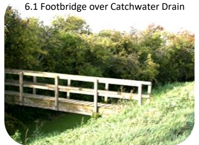
6.1 Footbridge over Catchwater Drain
